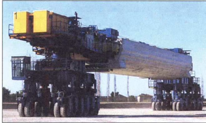
Figure 3 – The special launching crane transporting an omega beam to the viaduct.
